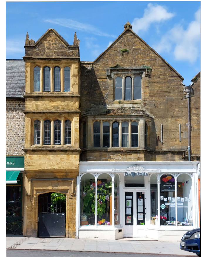
No 9 Fore Street, Chard, with a common entrance (left). Photo © P J Stow
